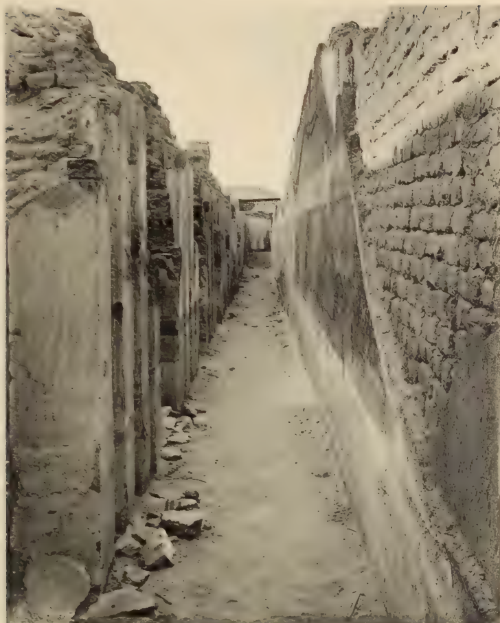
I. CORRIDOR FROM SOUTH.
